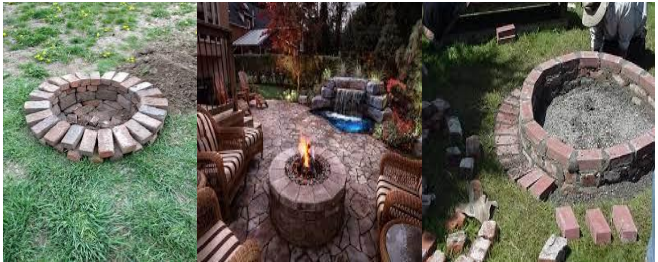
Fig.1 Construction of the Furnace
