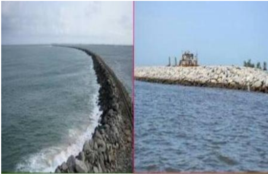
FIGURE 4. East and West mole breakwaters, Lagos Nigeria (Omar, 2017).
