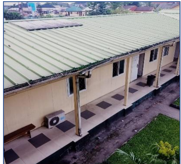
Figure 3.3 View showing roof with solar panel
