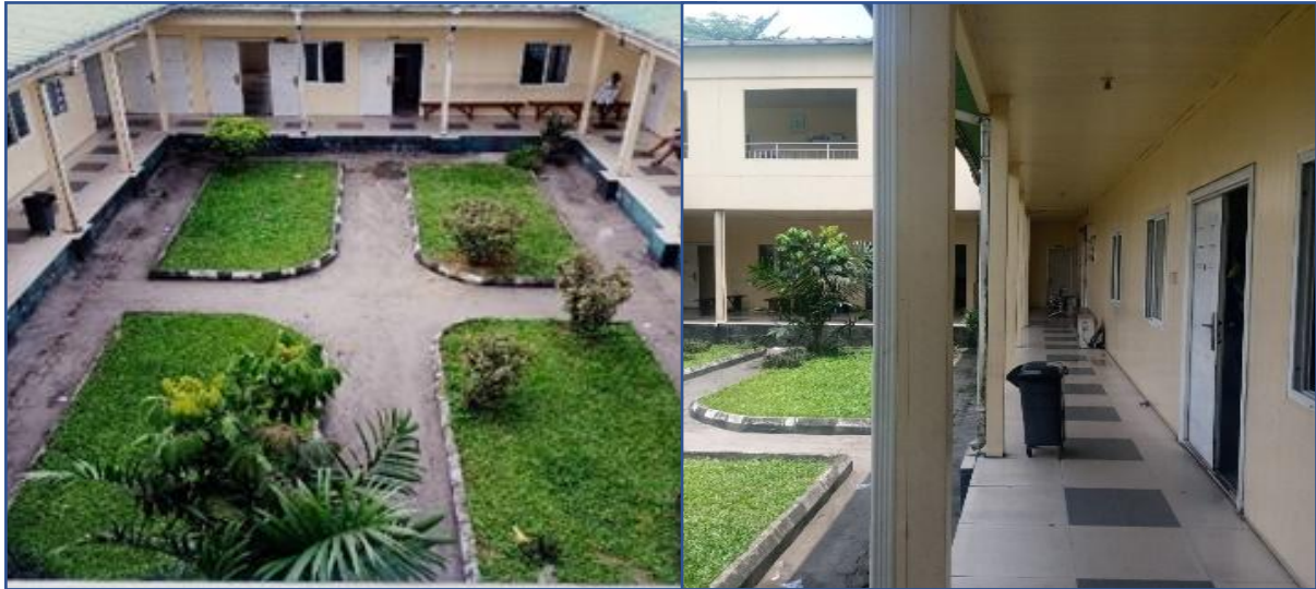
Figure 3.4 Courtyard Showing Wall finish with Poly-thane sandwich (metal sheet) panel with an insulating Poly-thane foam
